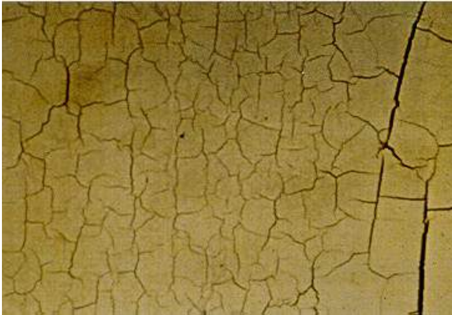
Figure 2.8.1(a) Checking
