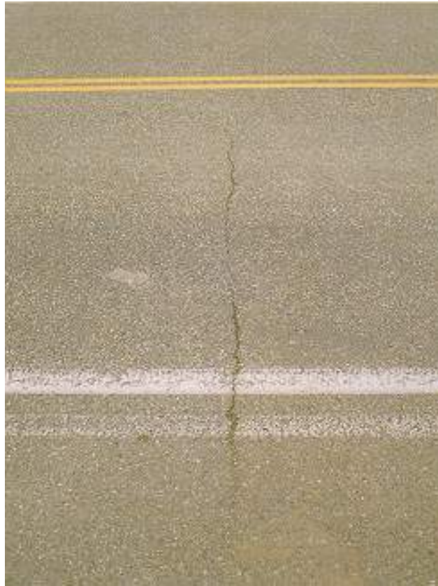
Figure 2.7.1(b) Medium Transverse Crack
