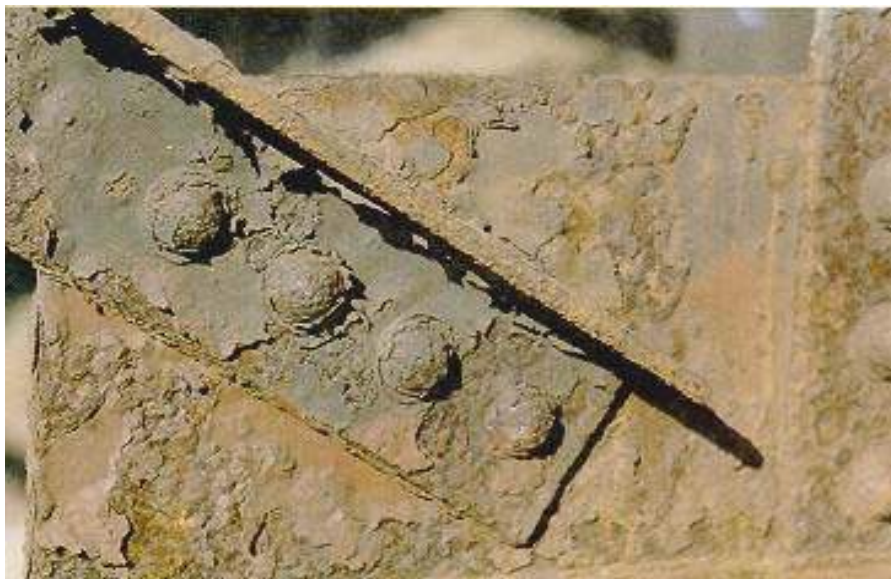
Figure 8.14(b) Sway Frame Connection.
