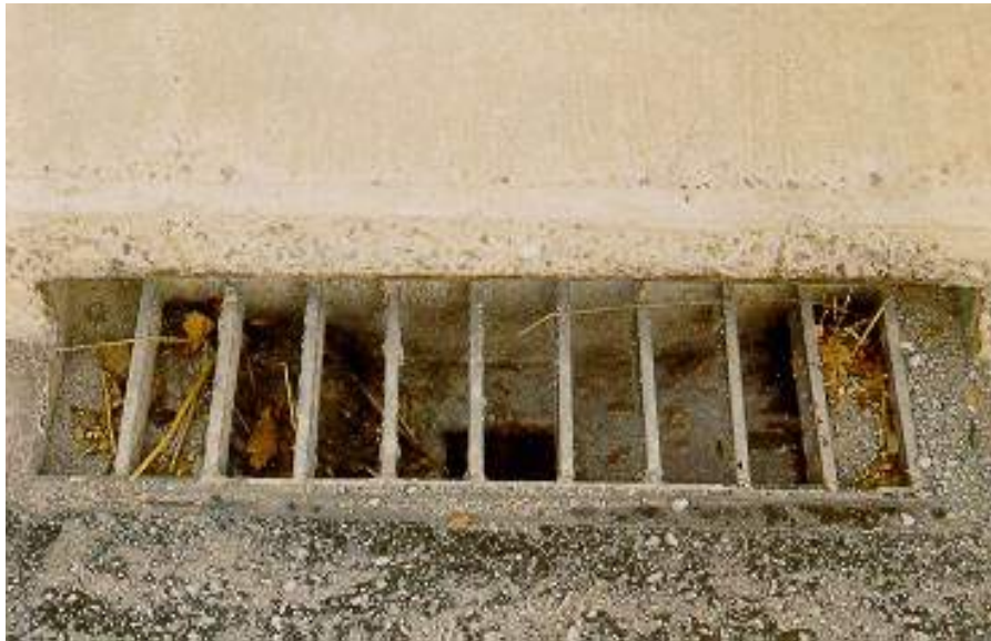
Figure 8.8(g) Deck Drain With Basin
