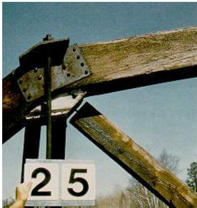
Figure 2.4.7 Loose Connection in Wood (25 mm gap measured)
