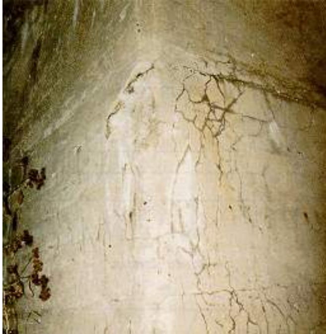
Figure 2.2.7(c) Medium Pattern Cracks in an Abutment
