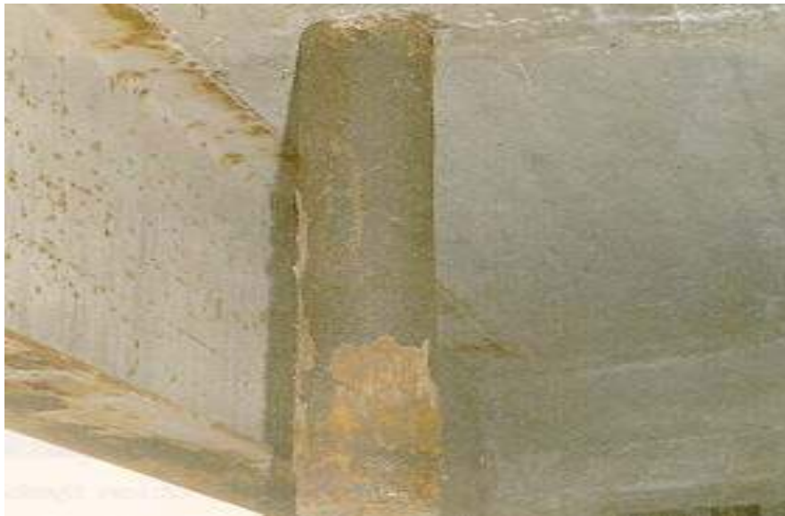
Figure 8.8(f) Steel Deck Drain
