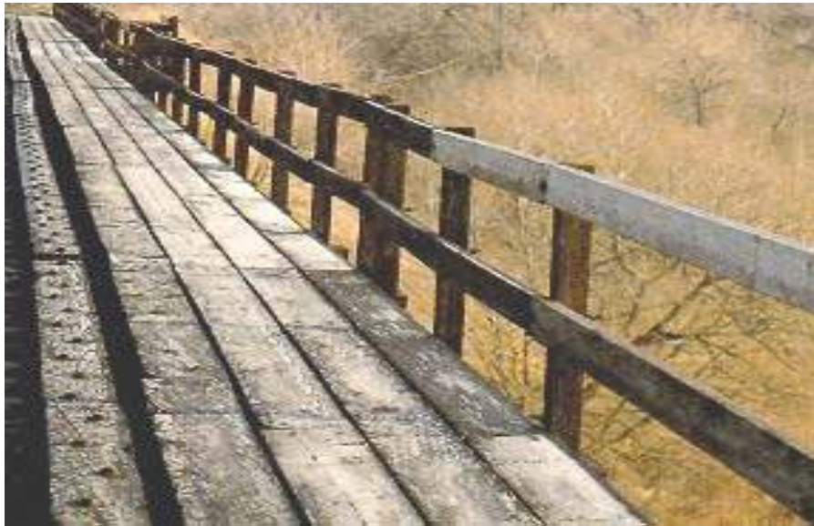
Figure 8.2(e) Wood Sidewalk
