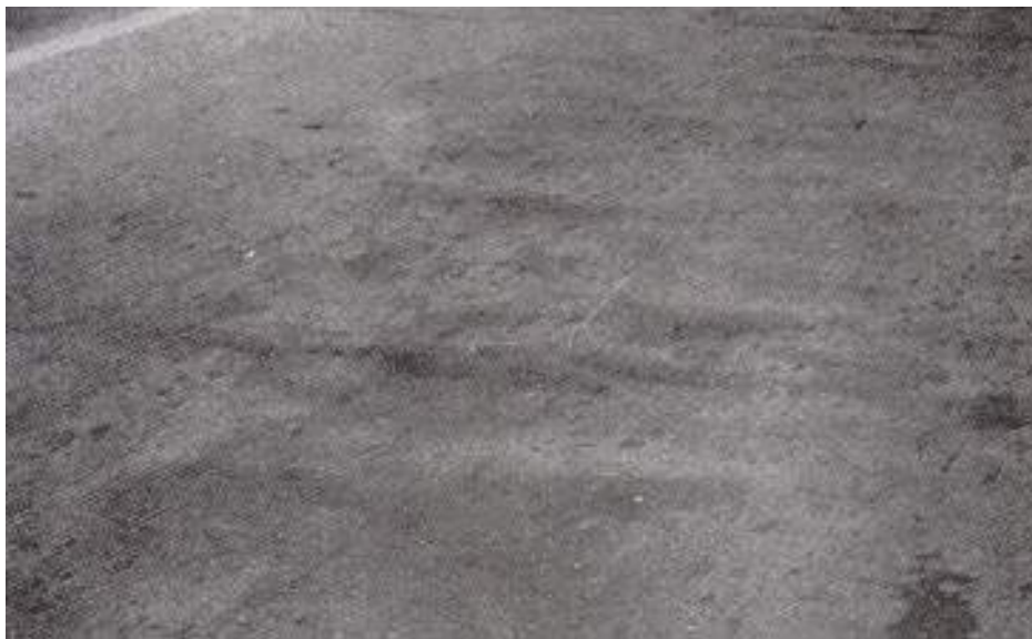
Figure 2.7.6 Severe Rippling
