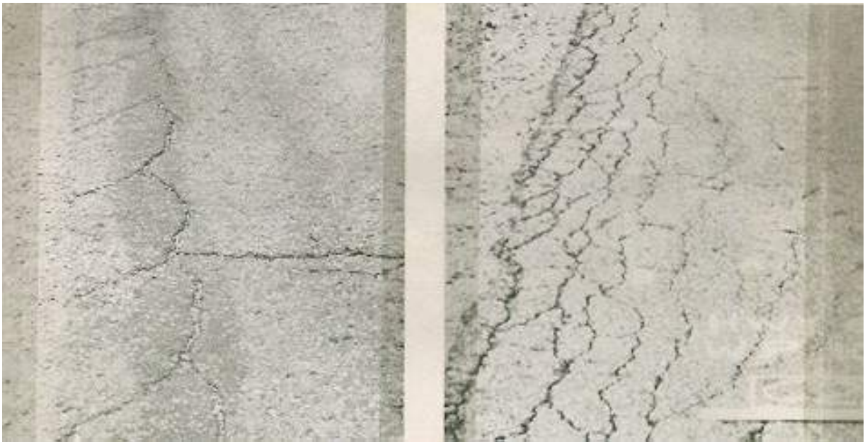
Figure 2.7.1(e) Medium Progressive Edge Cracks
