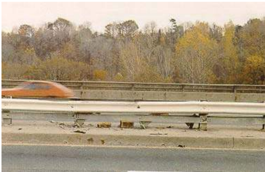
Figure 8.3(h) Steel Flex Beams
