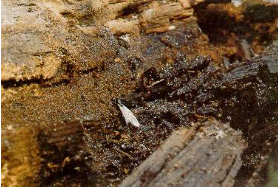
Figure 2.4.3(b) Very Severe Insect Damage in Wood
