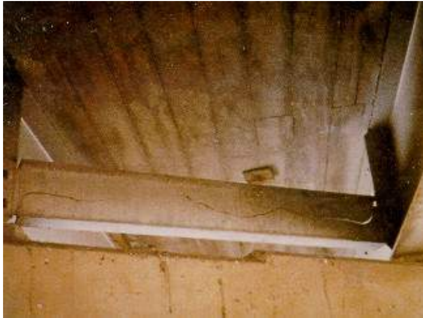
Figure 2.3.3(a) Very Wide Cracks in a Diaphragm
