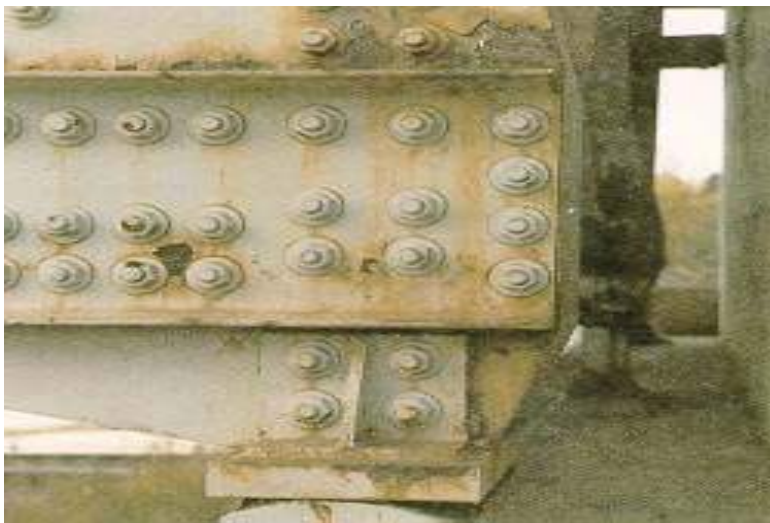
Figure 8.6(f) Truss Primary Connection at Abutment Bearing
