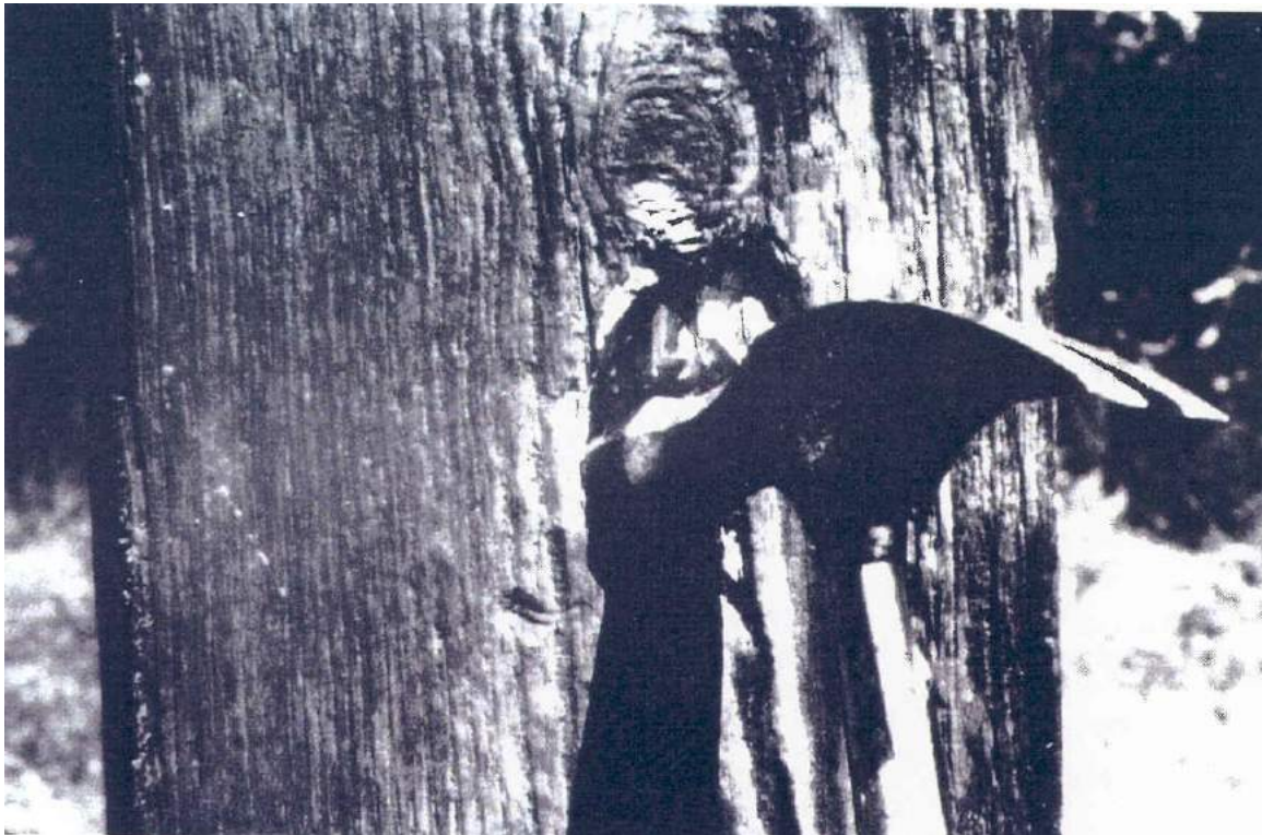
Figure 2.3.2 Simple use of a hammer to sound a wood timber. Decay is indicated by a hollow sound.
