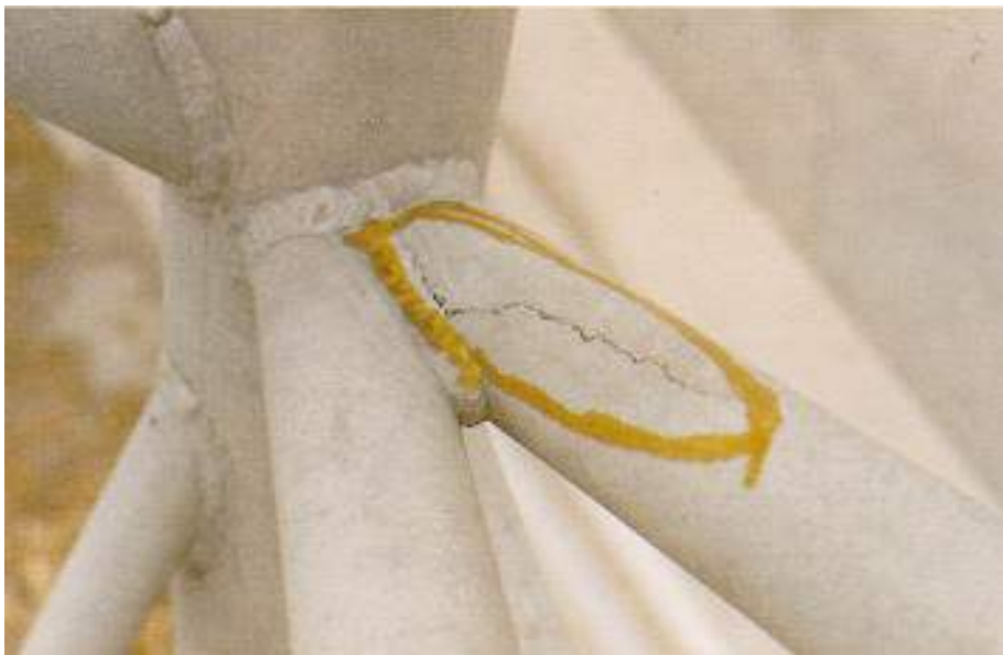
Figure 2.6.2 Wide Crack
