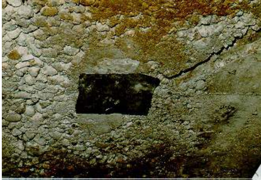
Figure 2.2.9 Severe Honeycombing in the Underside of a Deck Slab
