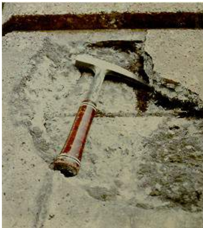
Figure 2.2.6(b) Severe Local Spalling
