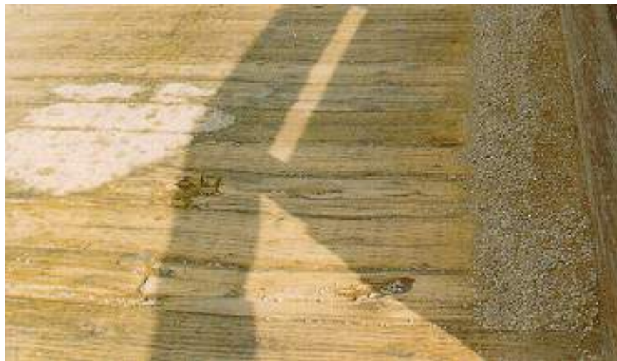
Figure 2.4.4(a) Very Severe Wear in a Wood Deck
