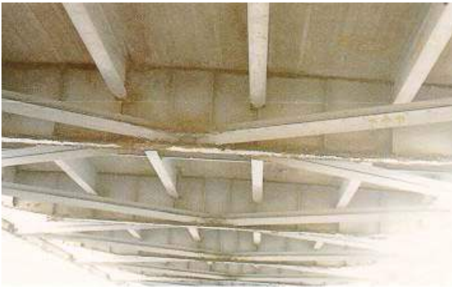
Figure 8.5(b) Bottom Lateral Bracing
