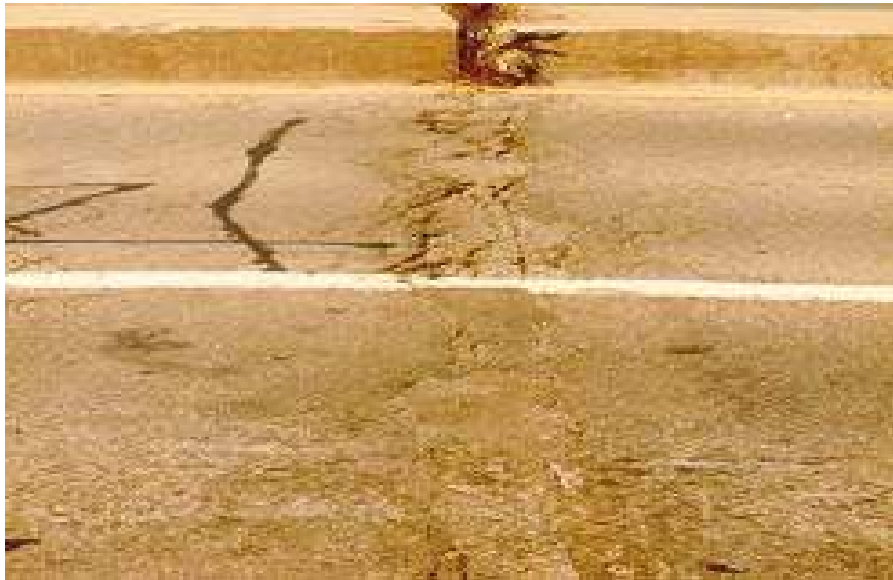
Figure 8.11(c) Paved-Over Joint
