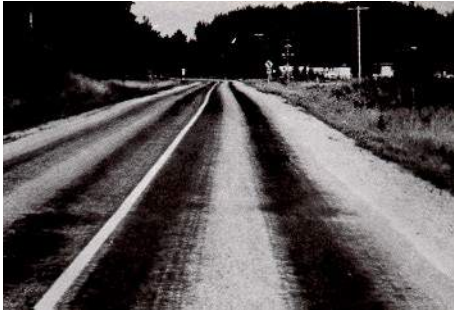
Figure 2.7.8 Slippery Surface
