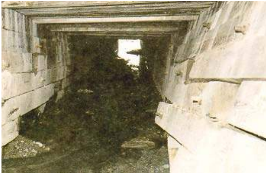
Figure 8.7(c) Wood Culvert
