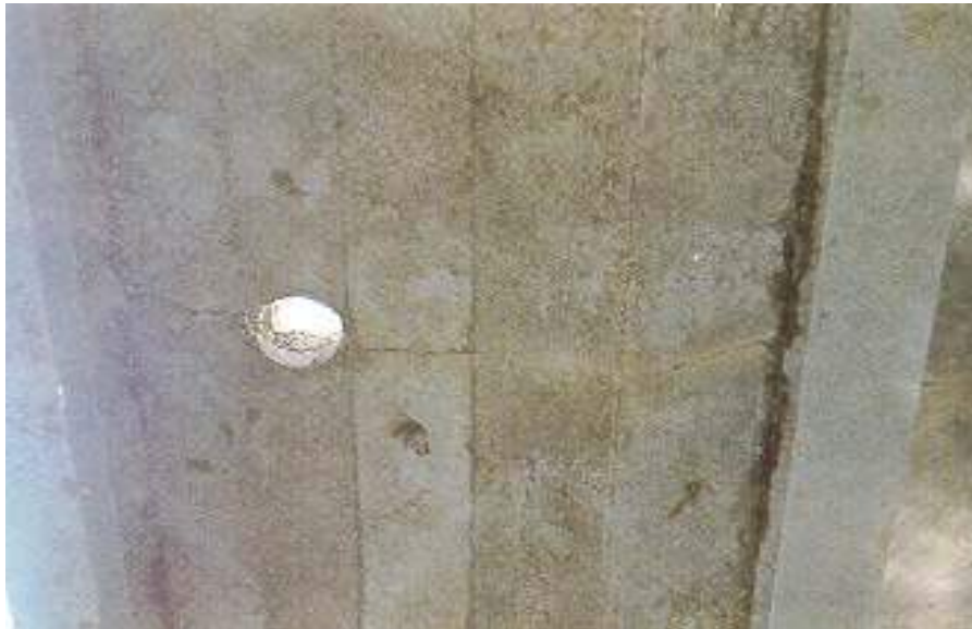
Figure 8.8(e) Deck Drain (Hole in Deck)
