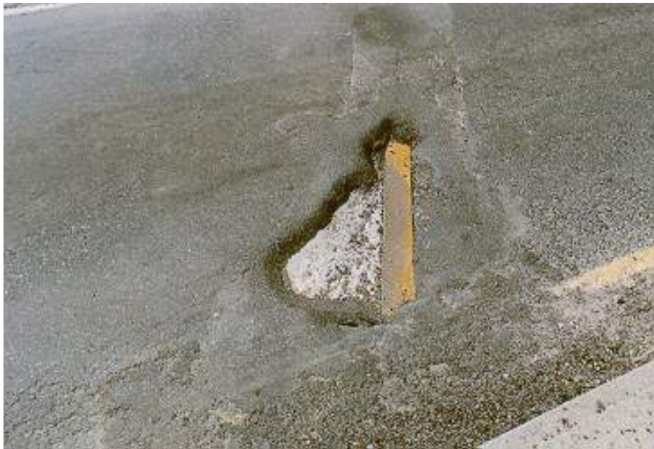
Figure 2.7.4 Severe Pothole
