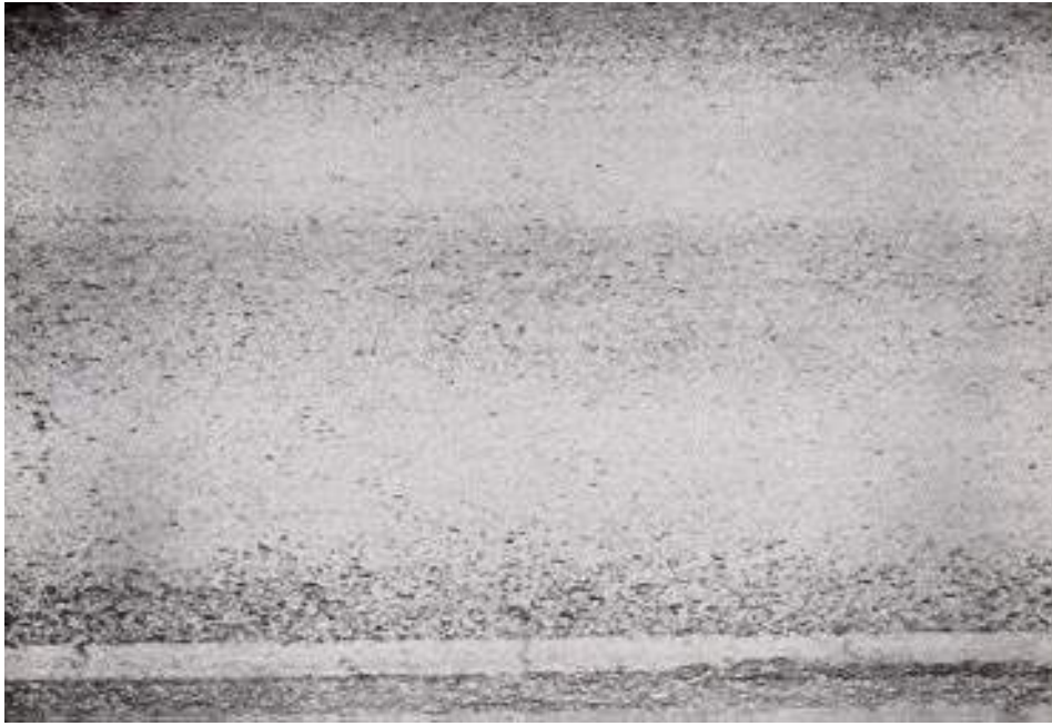
Figure 2.7.7 Severe Flushing
