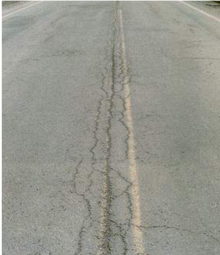
Figure 2.7.1(a) Medium Longitudinal Crack
