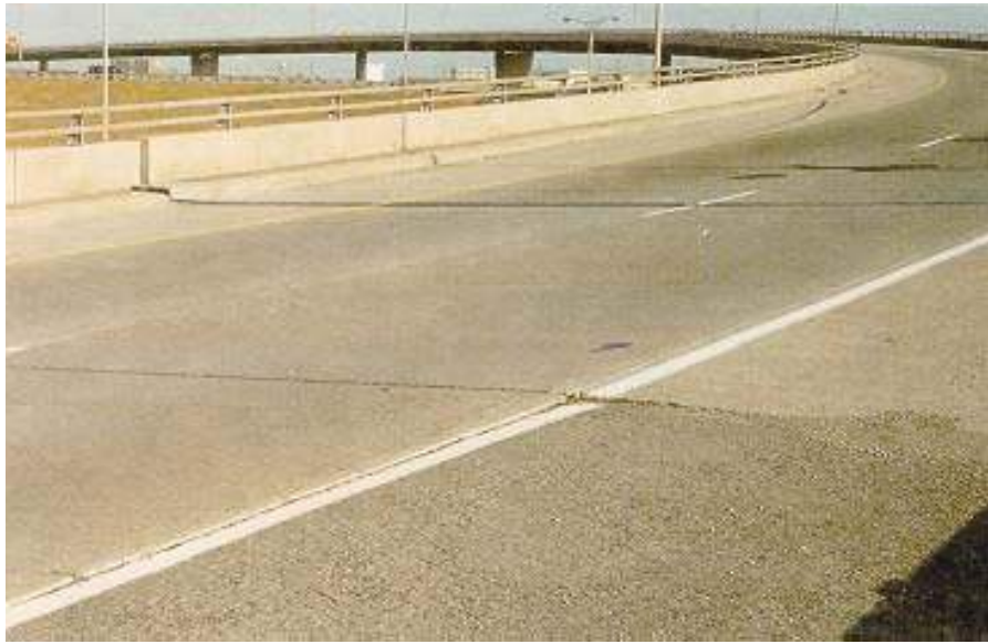
Figure 8.2(a) Concrete Approach Slab
