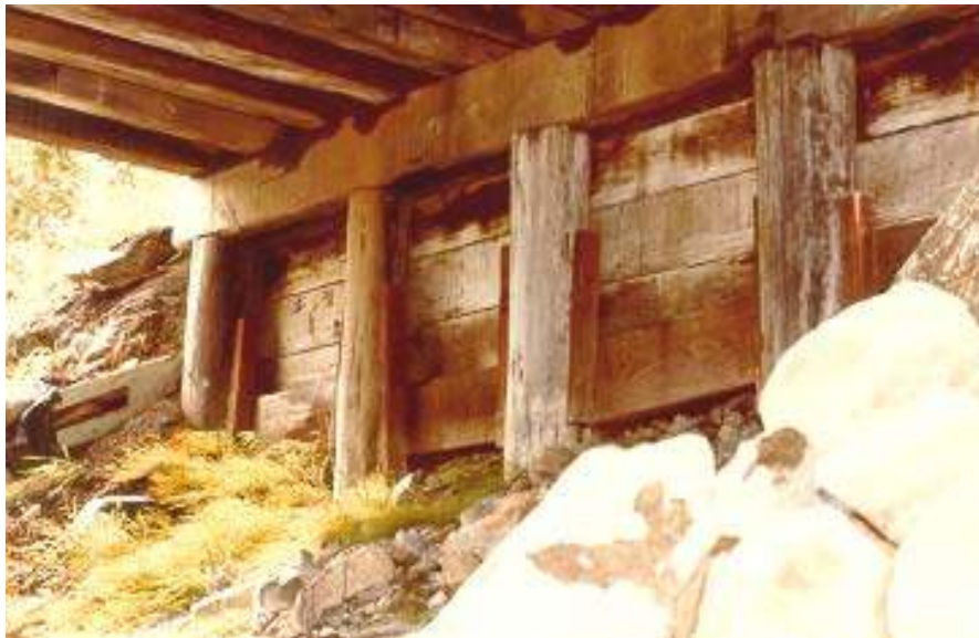
Figure 8.1(b) Wood Lagging - Abutment Wall
