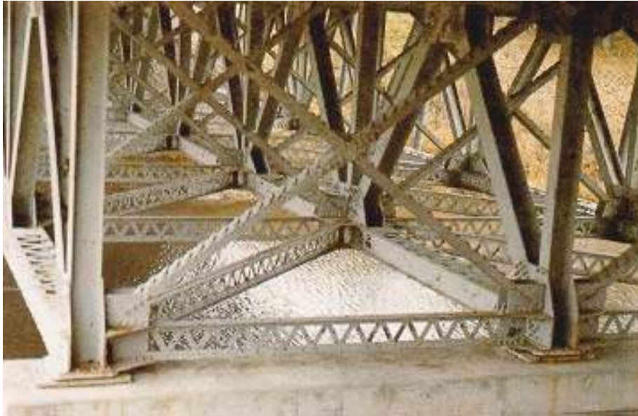
Figure 8.5(a) Sway Bracing and Bottom Lateral Bracing
