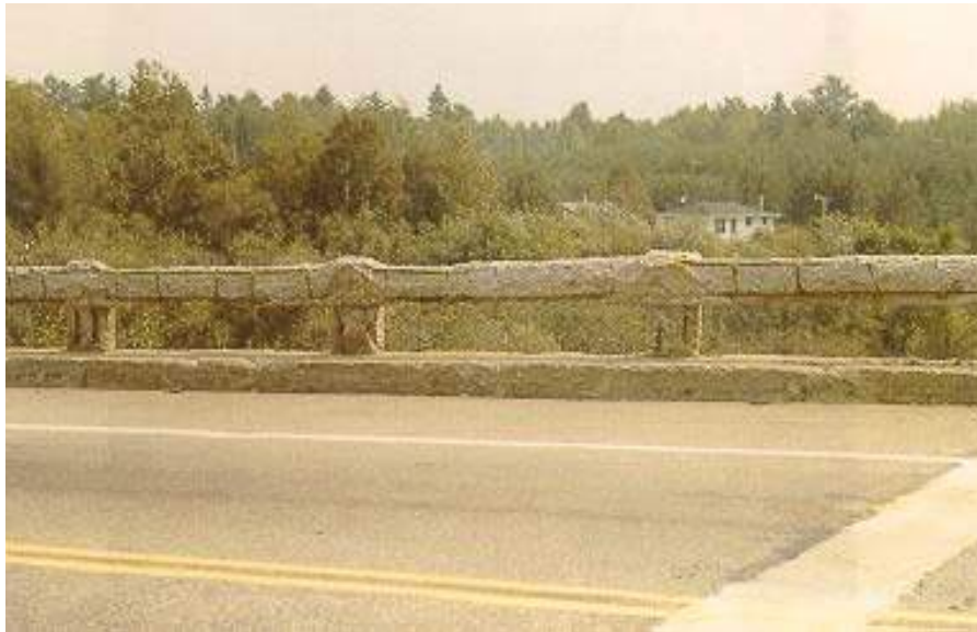
Figure 8.3(g) Concrete Guide Rail
