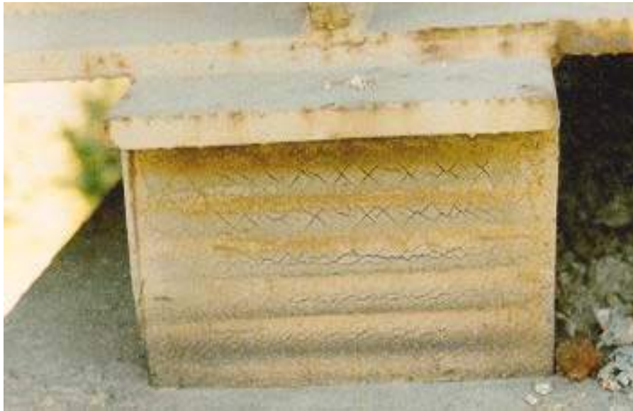
Figure 8.1(k) Laminated Elastomeric Bearing
