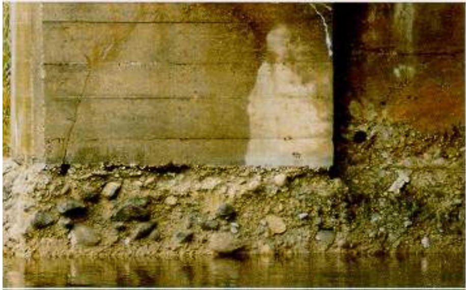
Figure 2.2.3 Very Severe Erosion of a Concrete Footing
