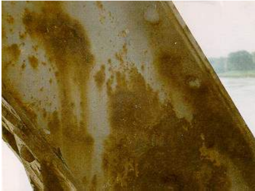
Figure 2.8.2(a) Undercutting
