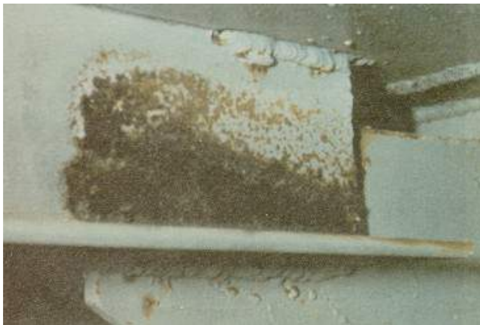
Figure 2.8.1(d) Chemical Attack
