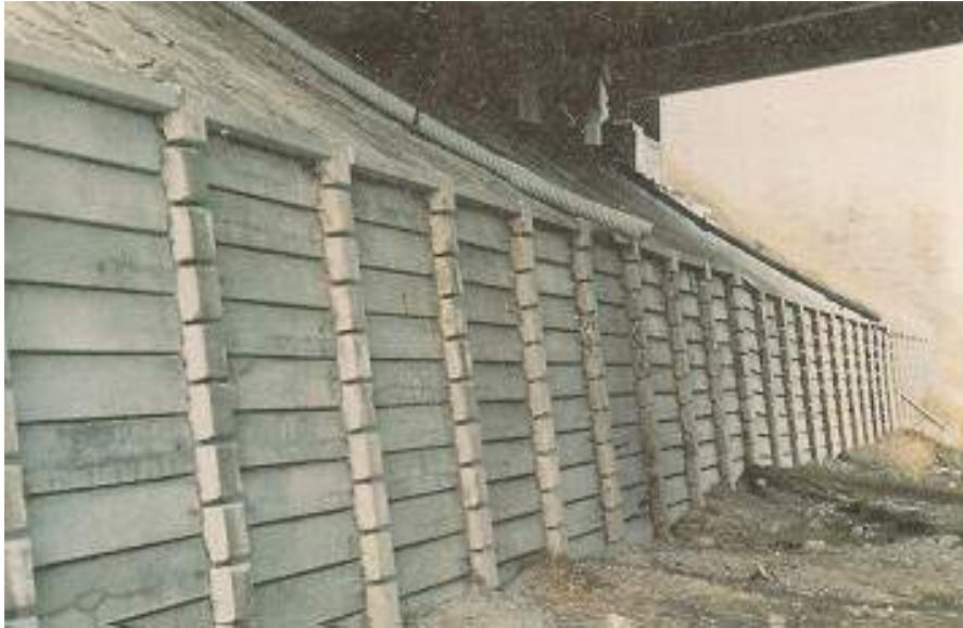
Figure 8.13(a) Precast Concrete Retaining Wall
