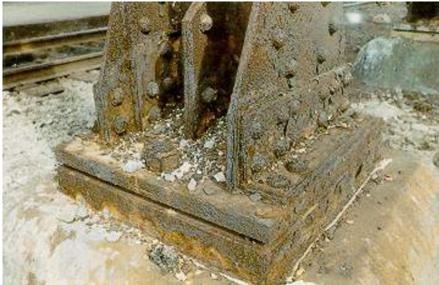
Figure 8.12(c) Steel Pier Bent Base
