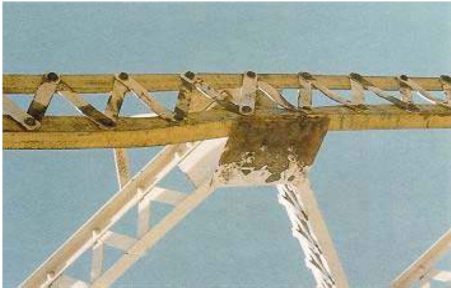
Figure 8.5(c) Top Lateral Bracing in Steel Through Truss
