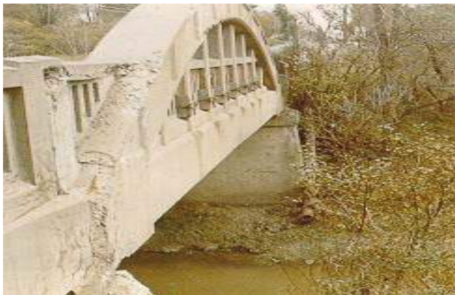
Figure 8.14(d) Concrete Bowstring Arch
