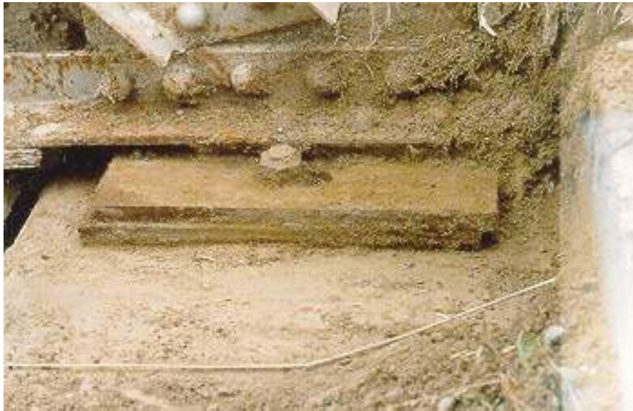
Figure 8.1(i) Steel Plate Sliding Bearing
