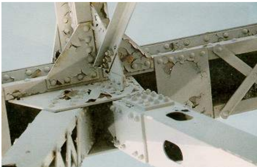
Figure 8.6(d) Through Truss - Connection of Primary Components
