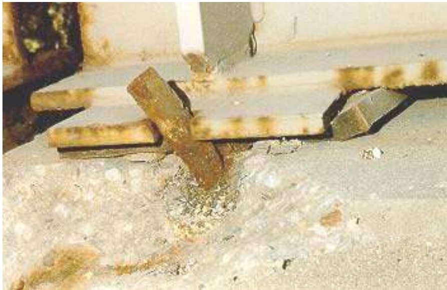
Figure 8.1(j) TFE Elastomeric Bearing
