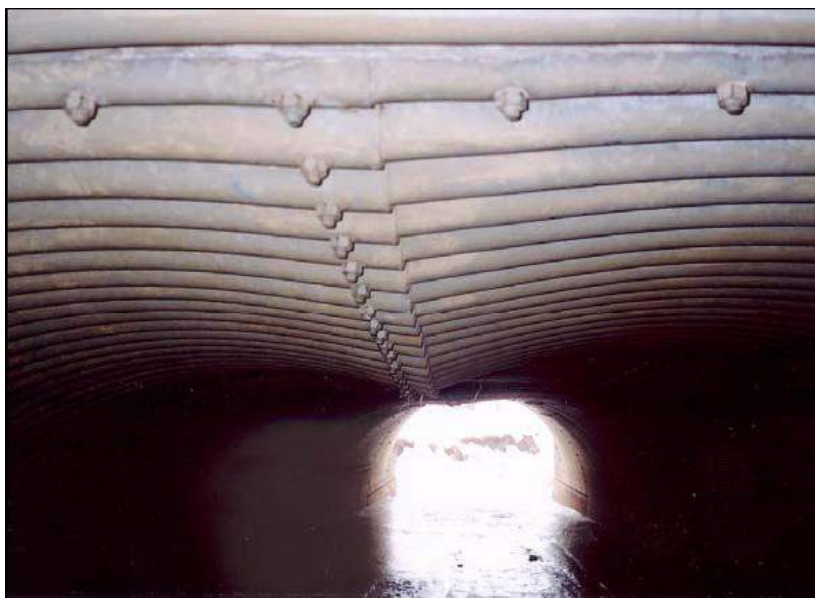
Figure 8.7(b1) Multi-plate Pipe Arch
