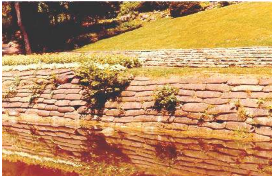
Figure 8.13(b) Bag Mortar Retaining Wall
