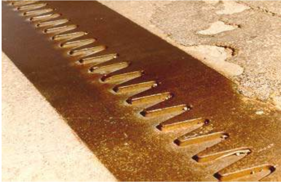
Figure 8.11(a) Finger Plate Expansion Joint
