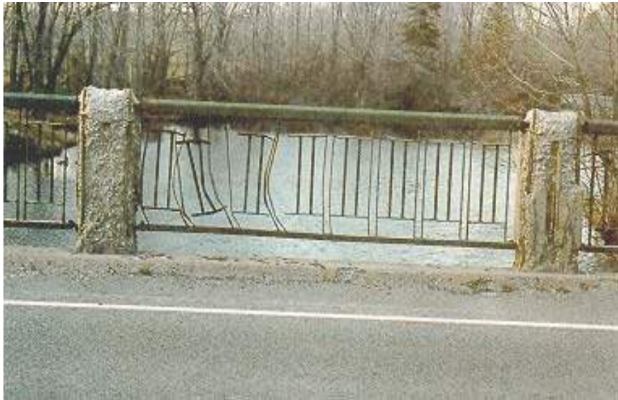
Figure 8.3(f) Steel Railing with Concrete Posts
