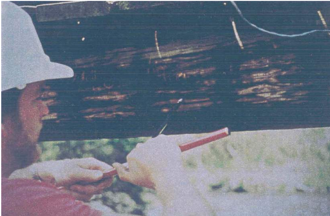
Figure 2.3.4b Simple application of the boring tool.
