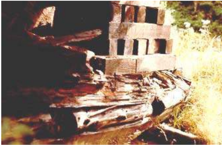
Figure 8.1(c) Wood Crib - Abutment Wall
