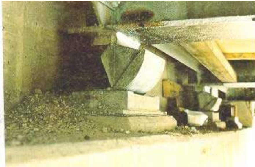
Figure 8.1(n) Steel Rocker Bearing
