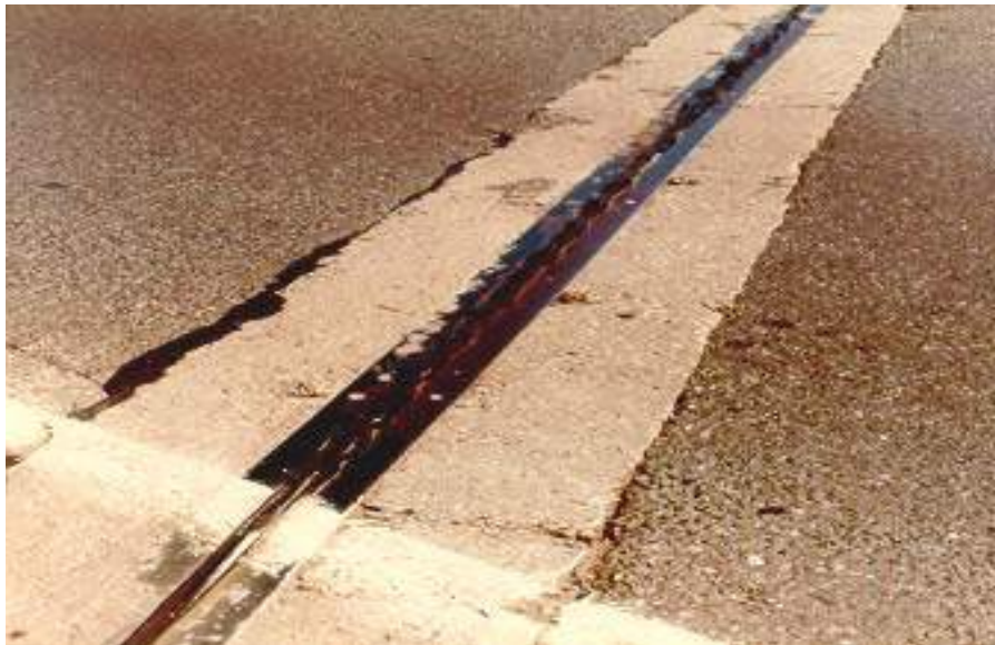
Figure 8.11(b) Compression Seal Joint
