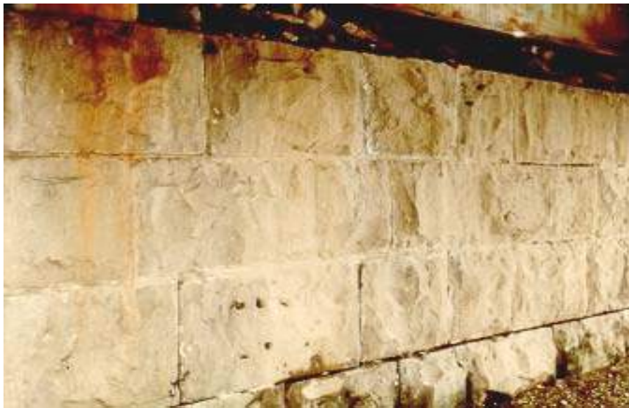
Figure 8.1(d) Masonry Abutment Wall
