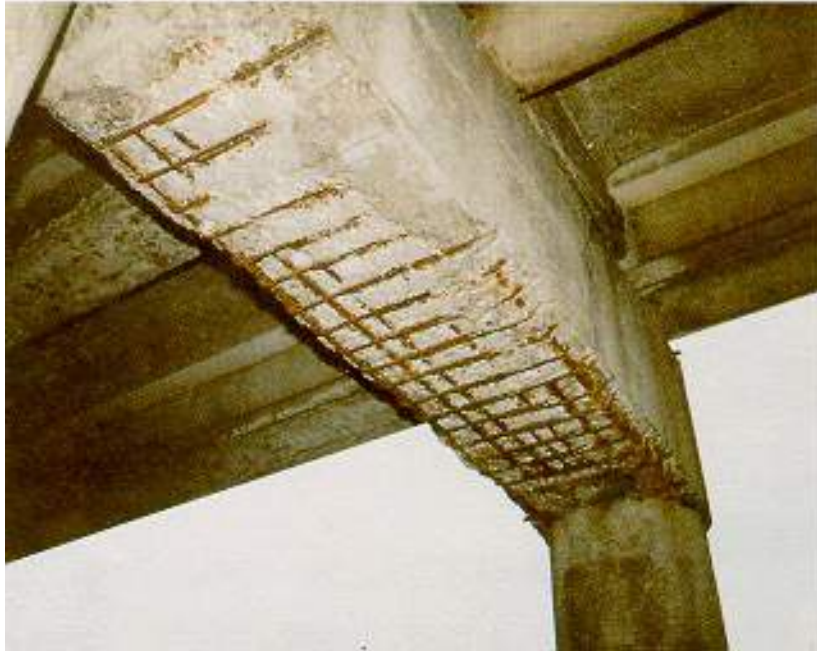
Figure 2.2.6(a) Very Severe Spalling in a Concrete Pier Cap Due to Corrosion of Reinforcement
