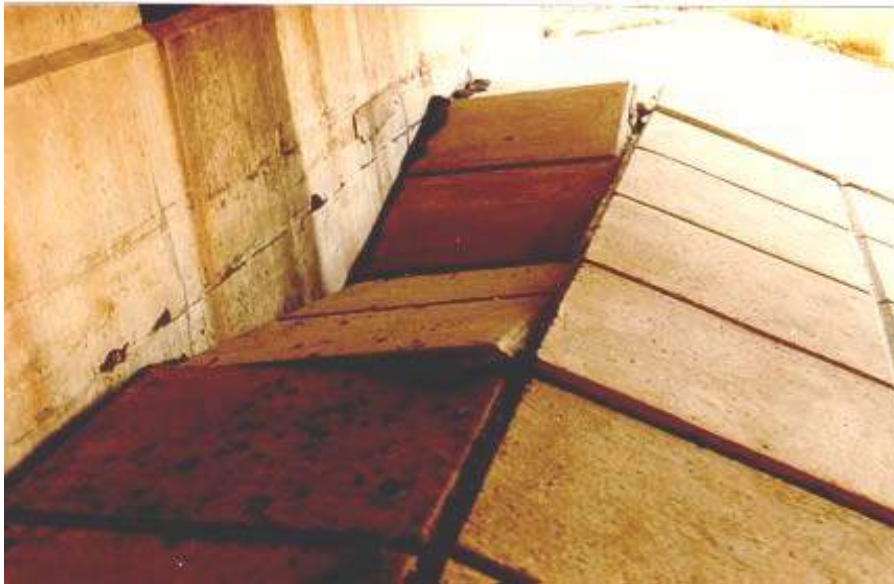
Figure 8.9(f) Cast-In-Place Concrete Slope Protection
