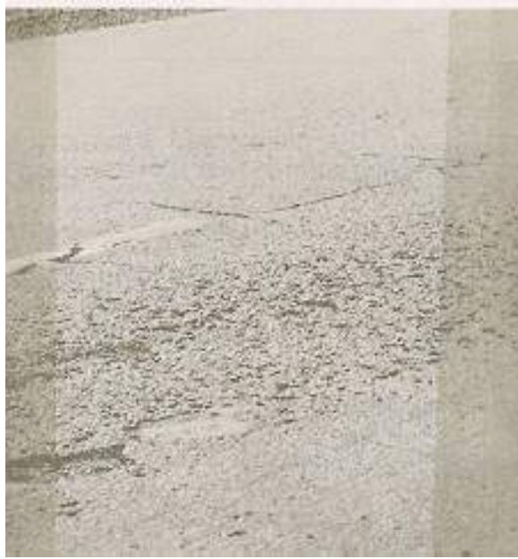
Figure 2.7.2 Severe Ravelling
