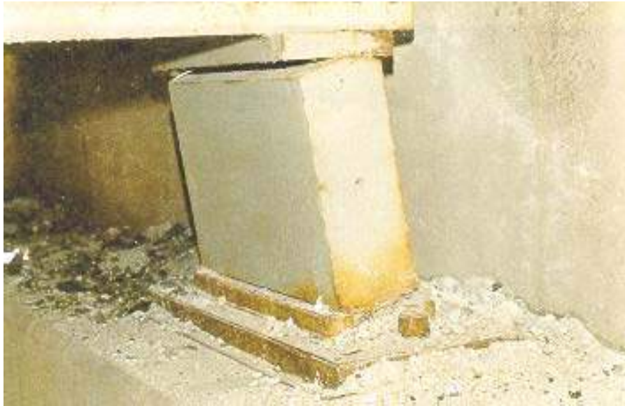
Figure 8.1(m) Steel Rocker Bearing
