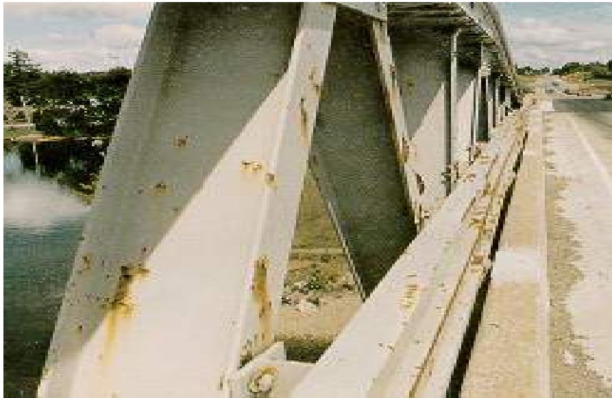
Figure 8.6(e) Steel Pony Truss
