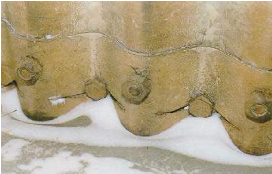
Figure 8.7(b) Multi-plate Pipe Arch
