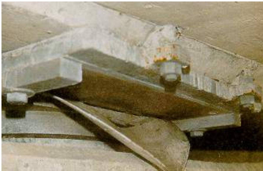
Figure 8.1(l) Pot Bearing
