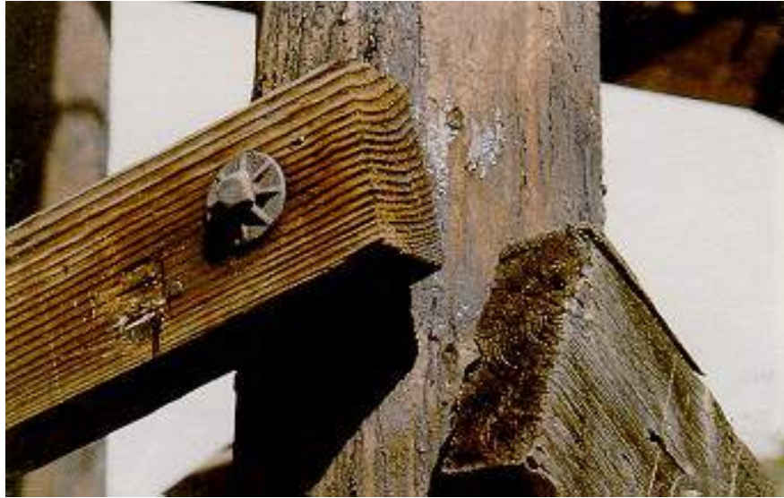
Figure 2.4.1(a) Light Weathering in Wood Members
