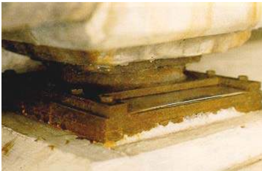
Figure 8.12(f) Disc Bearing
