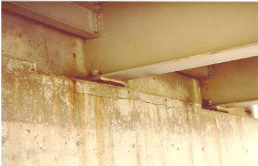
Figure 8.1(e) Concrete Abutment Wall
