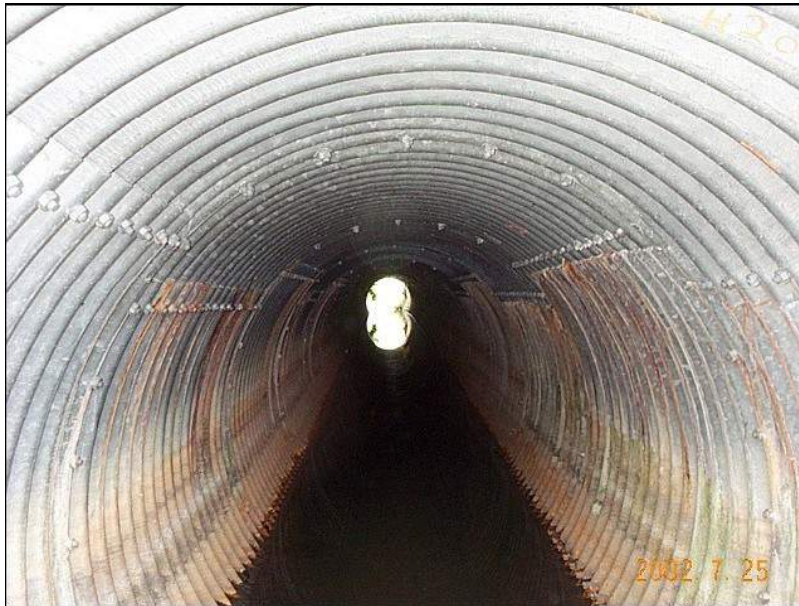
Figure 8.7(b3) Multi-plate Pipe Arch
