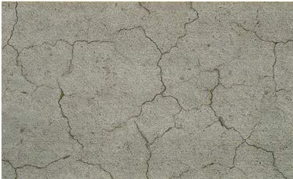
Figure 2.2.8 Severe Alkali-Aggregate Reaction
