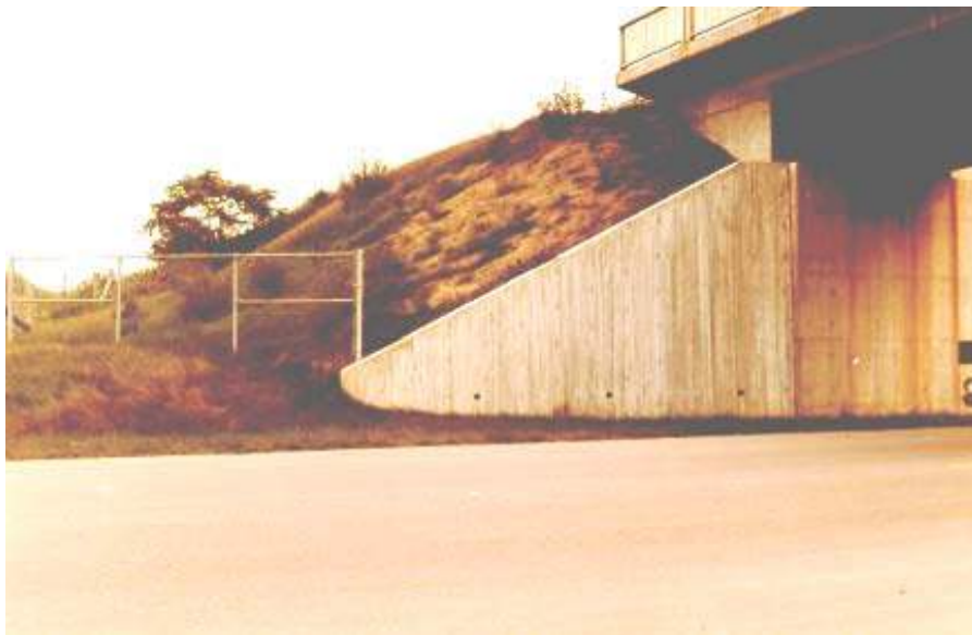
Figure 8.9(e) Grass Slope Protection
