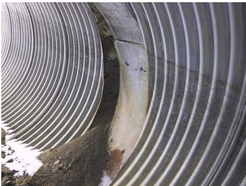
Figure 8.7(b2) Multi-plate Pipe Arch
