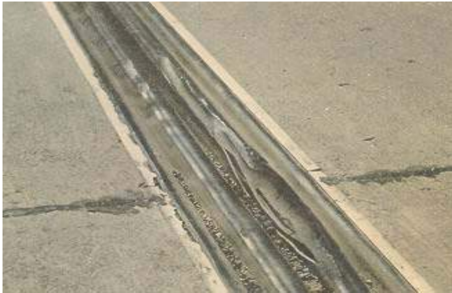
Figure 8.11(e) Multiple Seal Joint
