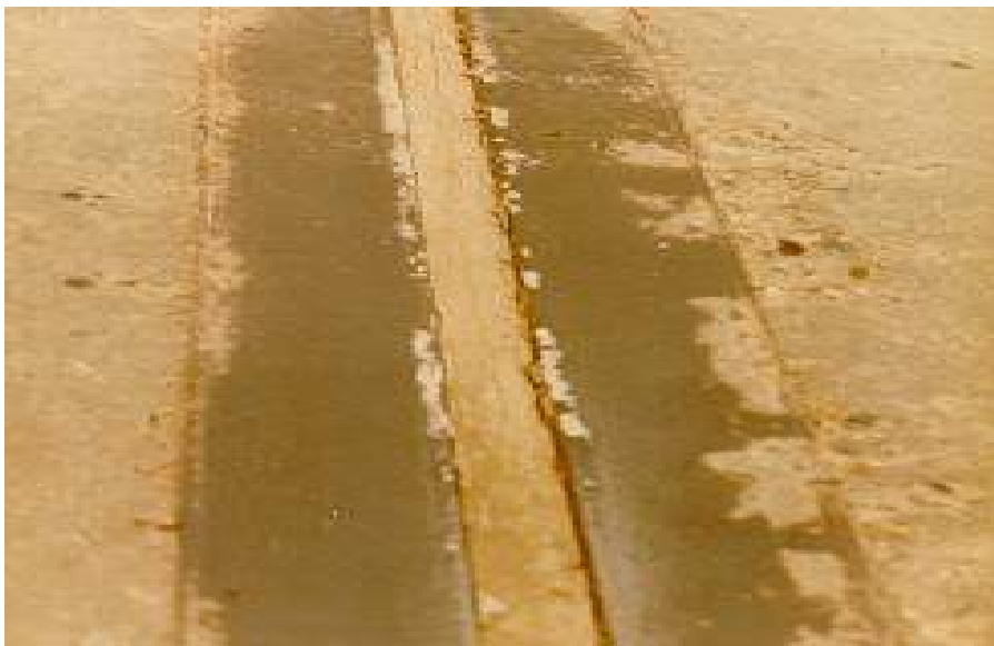
Figure 8.11(d) Ethylene Vinyl Acetate Seal
