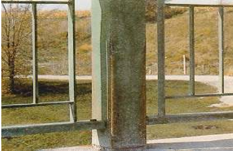
Figure 8.3(e) Steel Railing with Steel Posts (concrete filled)
