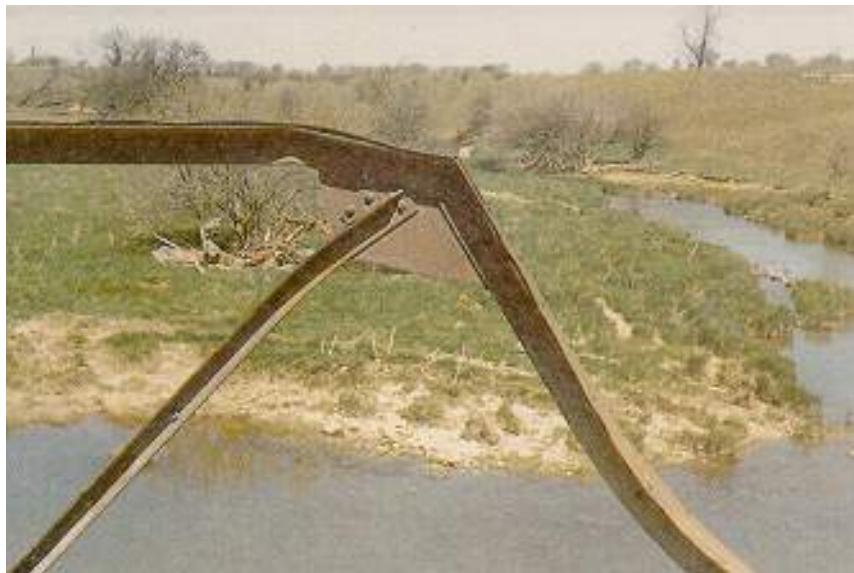
Figure 2.3.2 Very Severe Permanent Deformations by Impact
