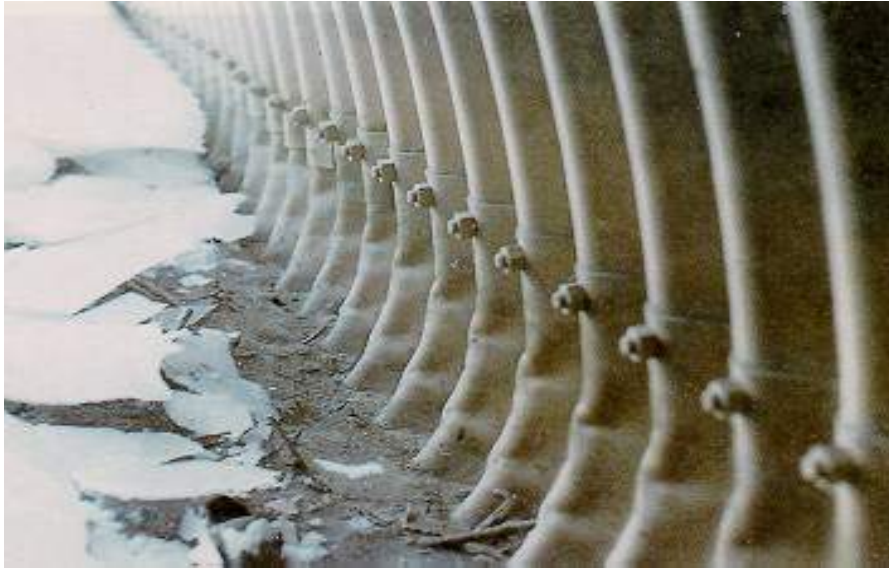
Figure 8.7(a) Multi-plate Pipe Arch
