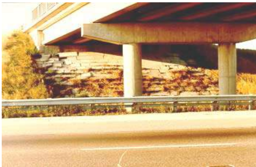
Figure 8.9(g) Precast Concrete Slope Protection
