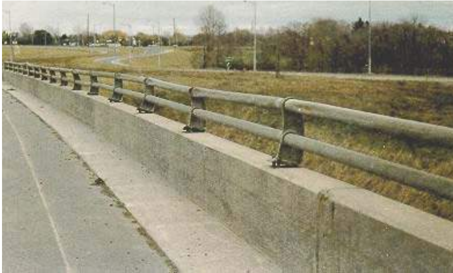
Figure 8.3(a) Parapet Wall
