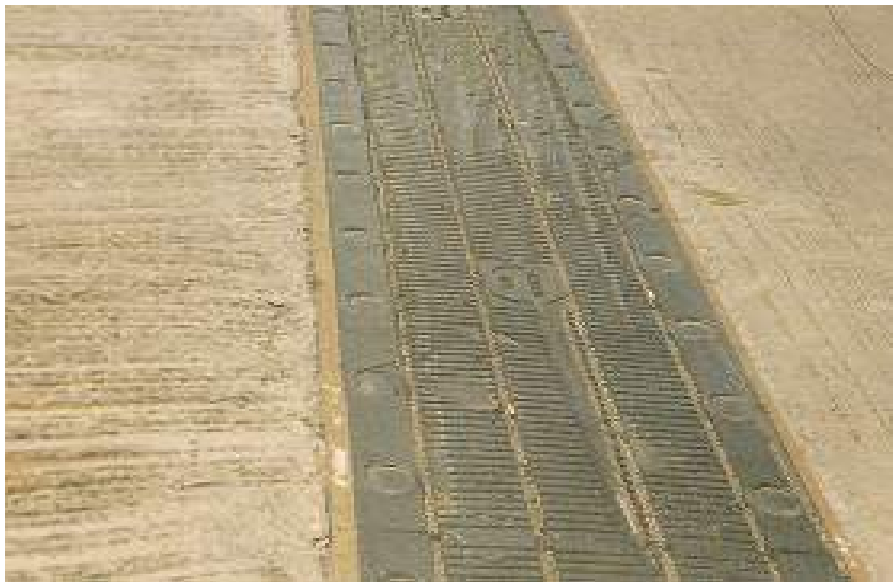
Figure 8.11(f) Rubber Cushion Joint
