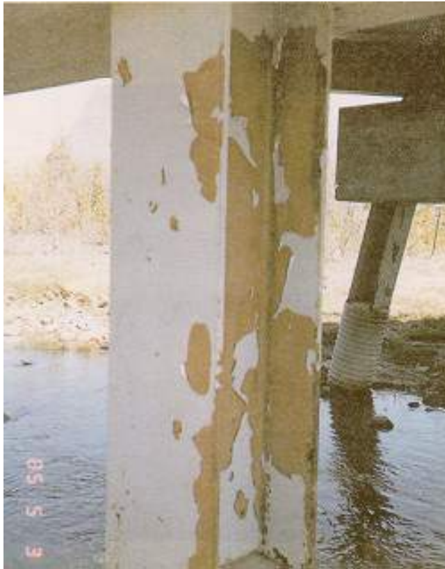
Figure 2.8.2(c) Intercoat Delaminations
