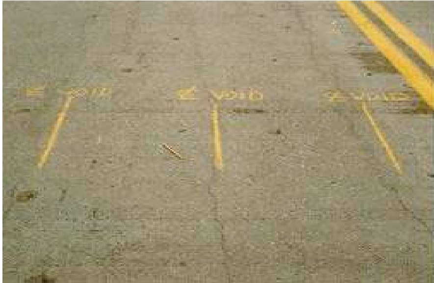
Figure 8.8(a) Exposed Concrete Deck of a Voided Slab
