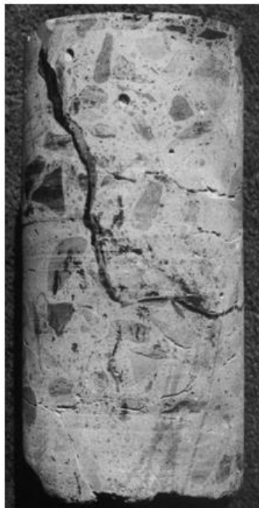
Figure 4.10 AAR-induced cracking representing a macrocrack, which may allow further deterioration to occur (core diameter 100 mm).
